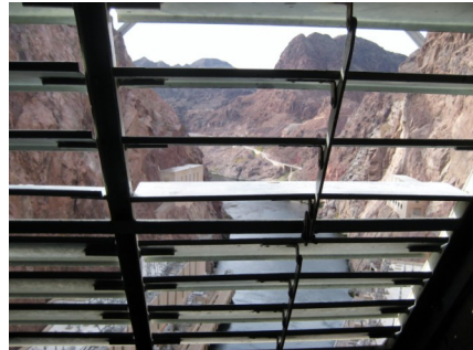
Fig. 3: Ventilation Grates with dam below
